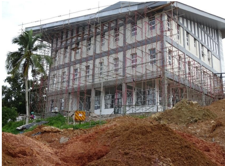
Construction of the administration building in progress
