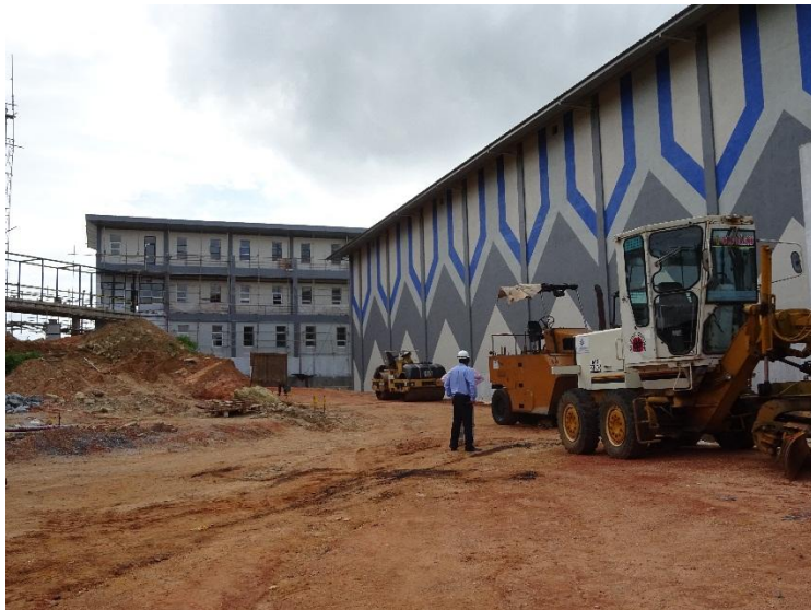
Landscaping around the laboratory building
