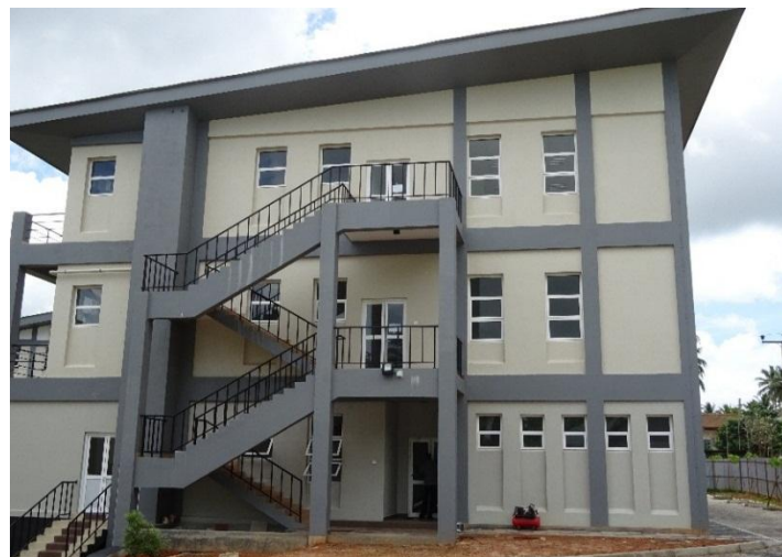
Phase 2 of the administration building – auditorium and legal metrology division
