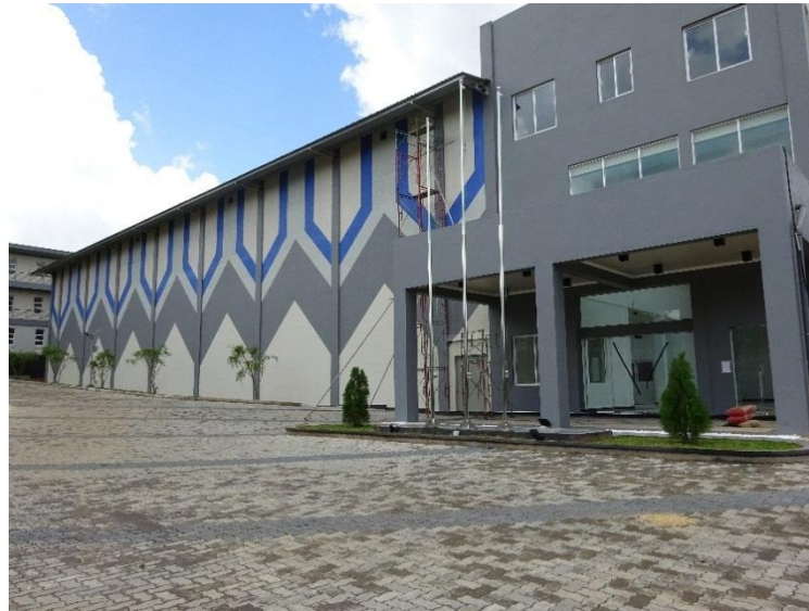
Completing constructions in front of the National Measurement Laboratory
